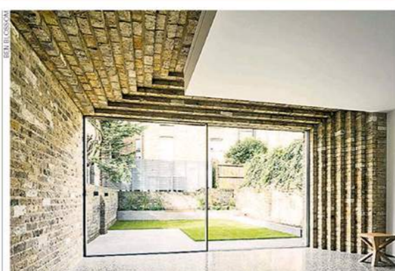
Bricks from the original back wall have been reused externally and internally to make this extension by the architects Bureau de Change feel integral to the house. Part of the extension roof is stepped, and this is reflected in the ceiling, with the bricks attached to steel beams.
