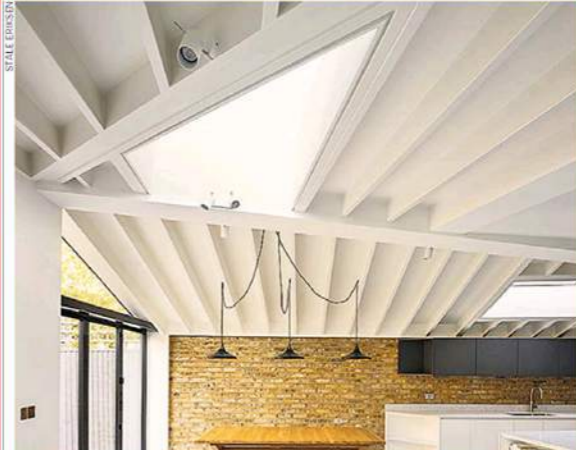
A desire to maximise width and height was the starting point for the ceiling in this extension by the architects Proctor & Shaw. A low, angled garden wall meant the site was wedge-shaped and the extension roof needed a steeper pitch on that side. The roof ridge rises towards the garden, so the rafters slope upwards. An angled roof light adds to the drama.
