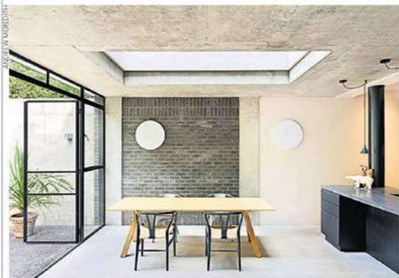
The concrete ceiling in this maisonette in a Victorian terrace helps to create the industrial look the owner wanted. The architects, Gundry & Ducker, supported the ceiling with pillars embedded in the walls. "Concrete ceilings need no maintenance and are great for soundproofing – you won't hear anyone walking about above," says Christian Ducker.
