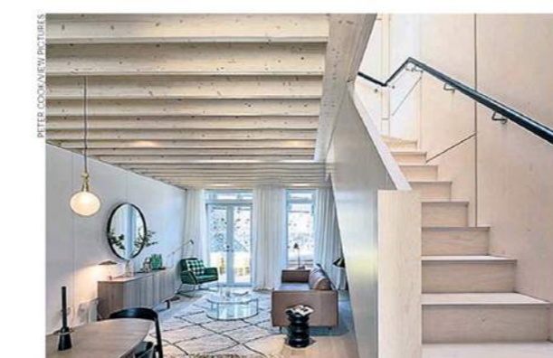
Leaving the ceiling cassette exposed in this low-cost modular house by the architecture and design studio TDO adds warmth and character, as well as increasing the ceiling height and allowing more light into the terraced home. It also reflects the birch-faced plywood staircase in the open-plan space.
