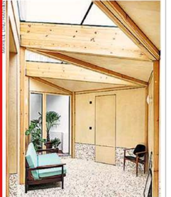
This extension to a flat in an octagonal former synagogue echoes the unusual geometry: triangular softwood ceiling sections alternate with triangular roof lights. "We transformed a dark, unused courtyard into a lofty, dynamic and unexpected space," says Sarah Castle, director of IF_DO architects.
