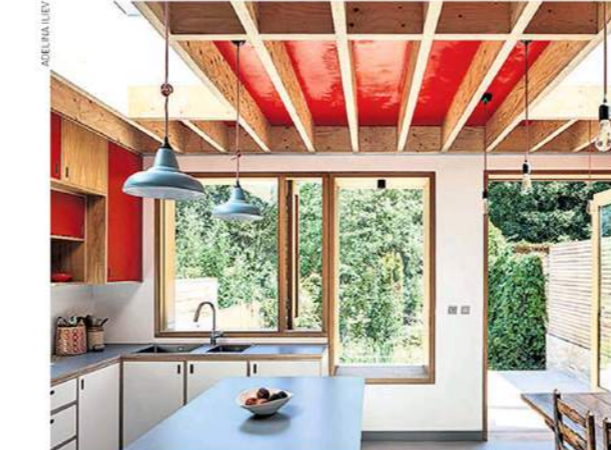
The structural timber of the ceiling in this extension has been left exposed, with sections in between painted red to match the wall units. "It makes the space vibrant and interesting, with the gloss finish bouncing light around the room," says the architect Catriona Burns.
